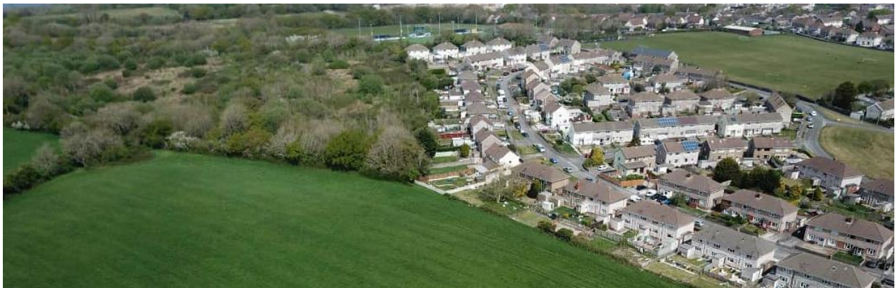
Figure 14 – Aerial view of the eastern boundary of the site and existing properties within Bryntirion
